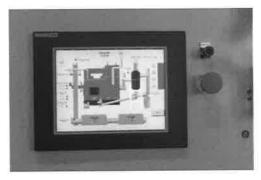
Biomass boiler controller integrates with the schools building automation system – and can be used for remote diagnostics.
