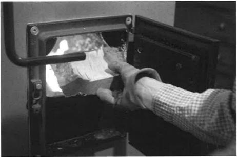
This 198,000-Btu/hr TARM cordwood boiler system, installed in 2008, heats the 6,000-square-foot dining hall at a mountain camp. Cold winters and cool summers at 10,000 feet above sea level keep the boiler going most of the year. The system cost about \$60,000 installed.
