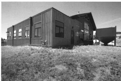
This 200,000-Btu/hr Froling P4 pellet boiler easily heats this 2,000-square-foot office building in Fort Collins, Colorado. The system is designed for bulk delivery of pellets, but the local market only offers bag delivery.
