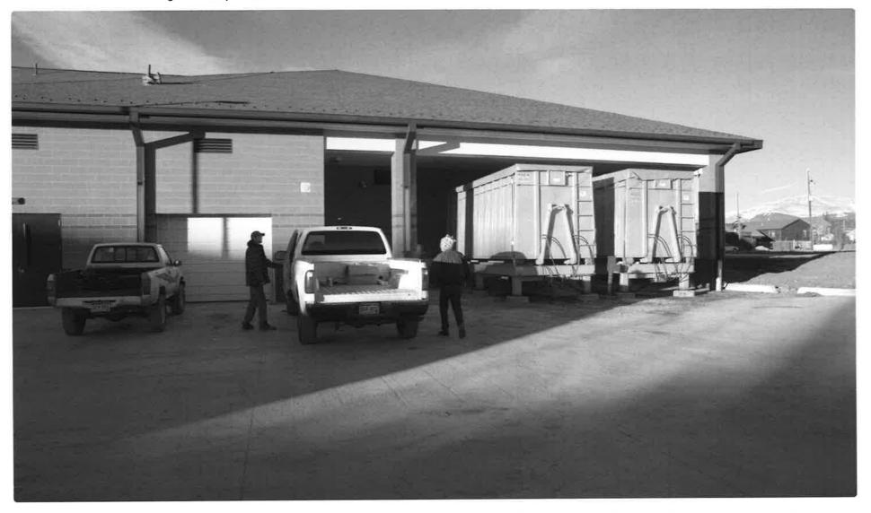
Chip container docking bay holds two containers, holding enough chips to heat the school for about 4 days during the coldest months.
