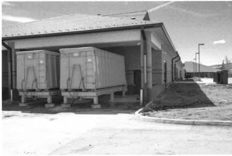
This 3.5-MMBtu/hr Osby Parca P500 wood chip boiler heats this LEED (Leadership in Energy and Environmental Design) certified school at 10,000 feet above sea level in Fairplay, Colorado. This system features an innovative chip bin and a rolloff container with a "walking floor" that automatically moves the chips to the end of the container and into the boiler's chip feeder. The system cost about \$500,000.
