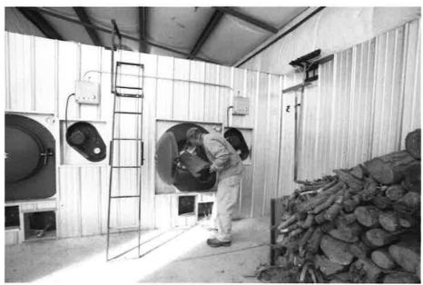
Two GARN WHS 2000 wood boilers can provide up to 850,000 Btu/hr when continuously fired (about every 2 to 3 hours). In typical operation, it has no trouble heating this recently renovated and winterized 18,000-square-foot mountain camp.
