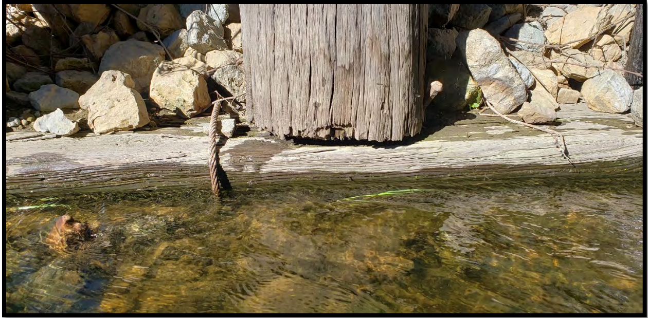
Column Deterioration Typical (South Pier Shown)
