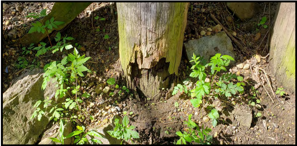
Pier 2-Pile Section Loss (upstream pile)
