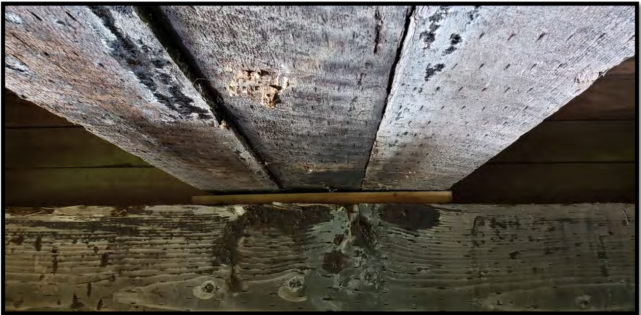
Gap-South Abutment (Wood “Shim” between Stringer and Column Cap)
