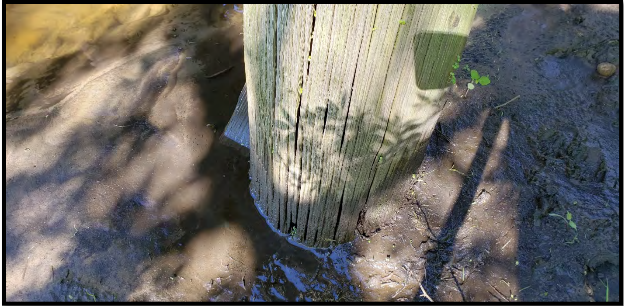
Pier 4-Pile Splits/Section Loss (upstream pile)
