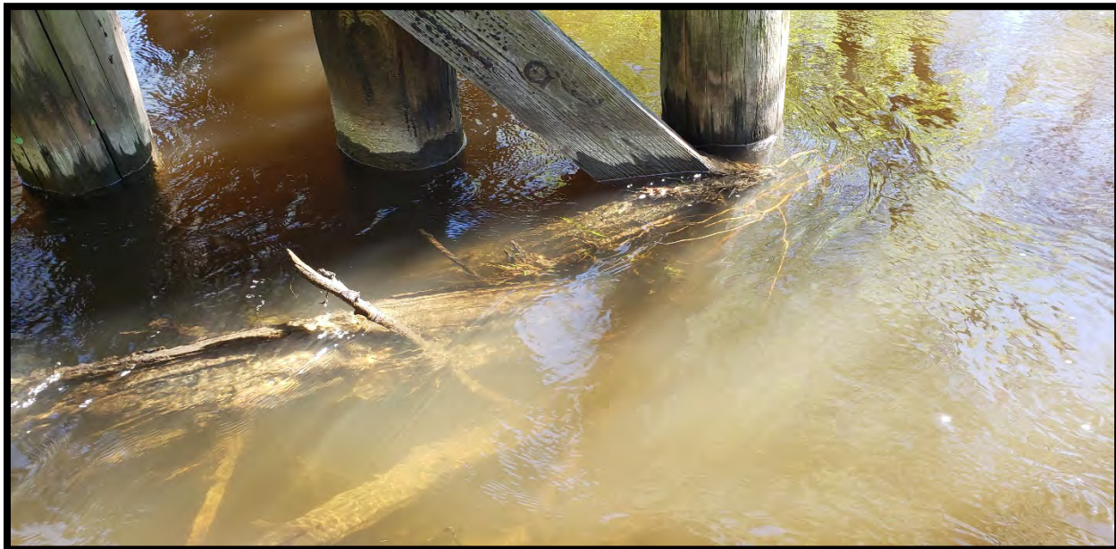
Pier 3-Upsteam flood debris
