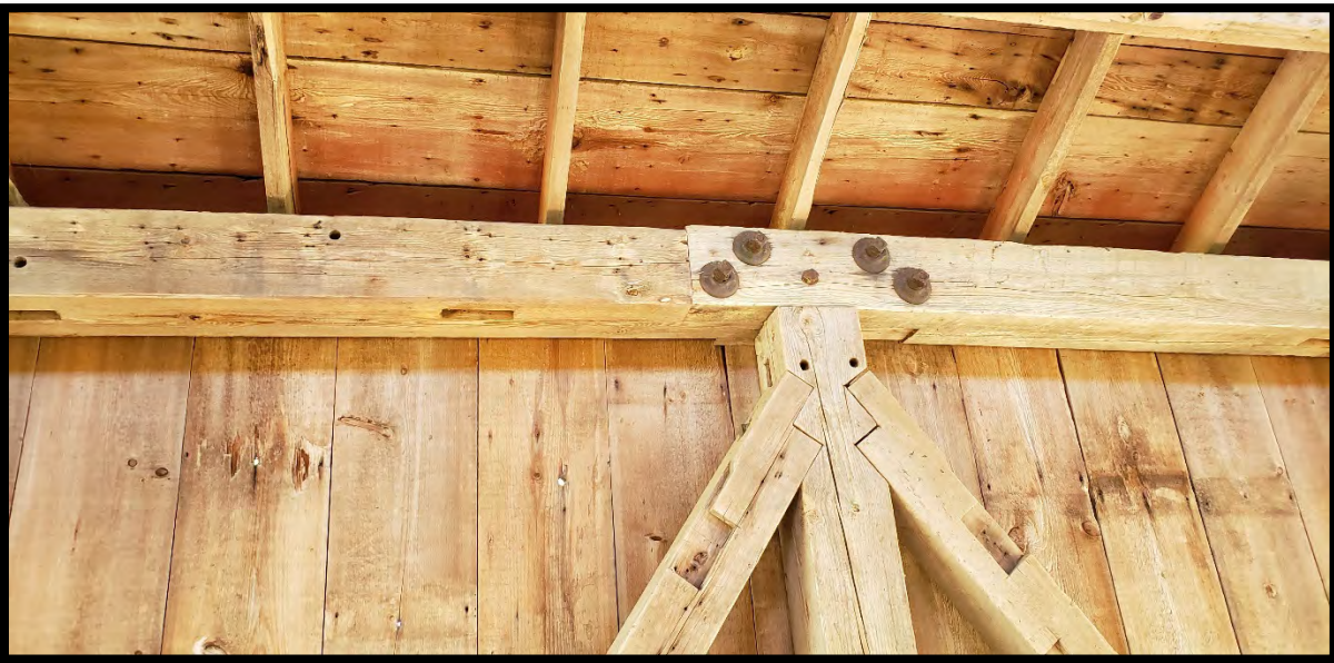
Superstructure-Timber beams and Trusses
