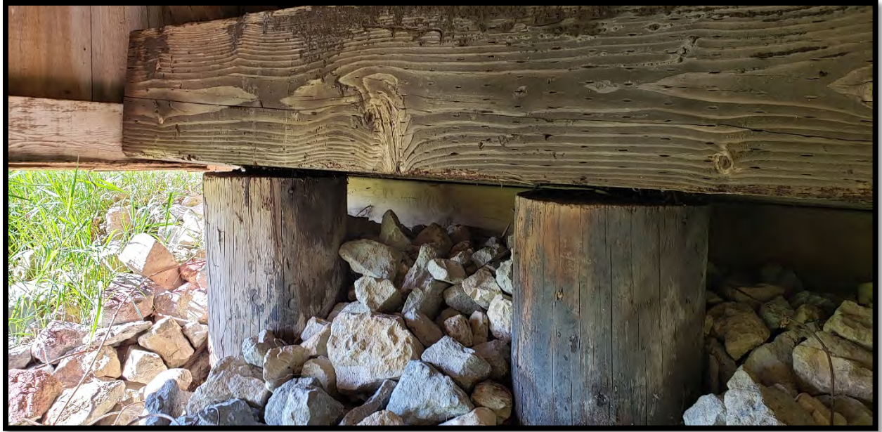
Gap-South Abutment (Between Column Cap and Columns-due to rotated cap)
