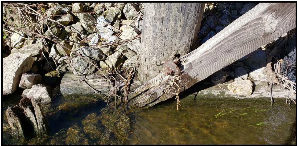
Pier Lateral Bracing-Broken Connection South Pier
