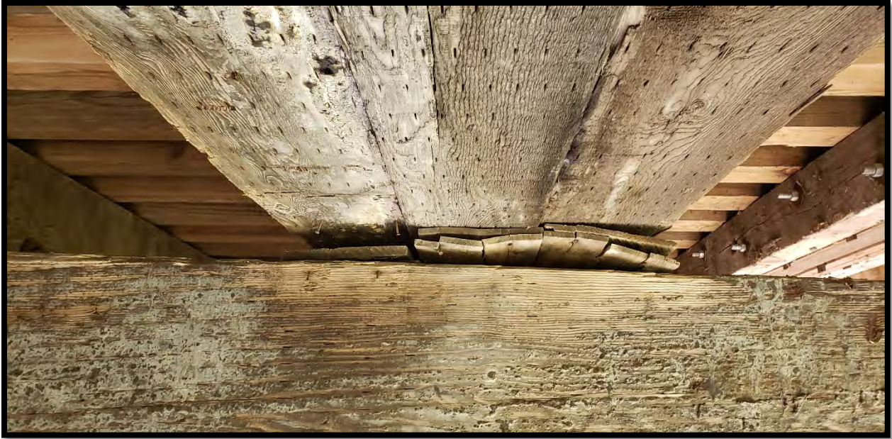
Gap-North Pier (Between Stringer and Column Cap)
