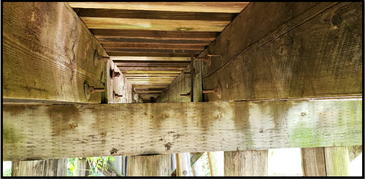
Timber Stringers and Floor Beams
