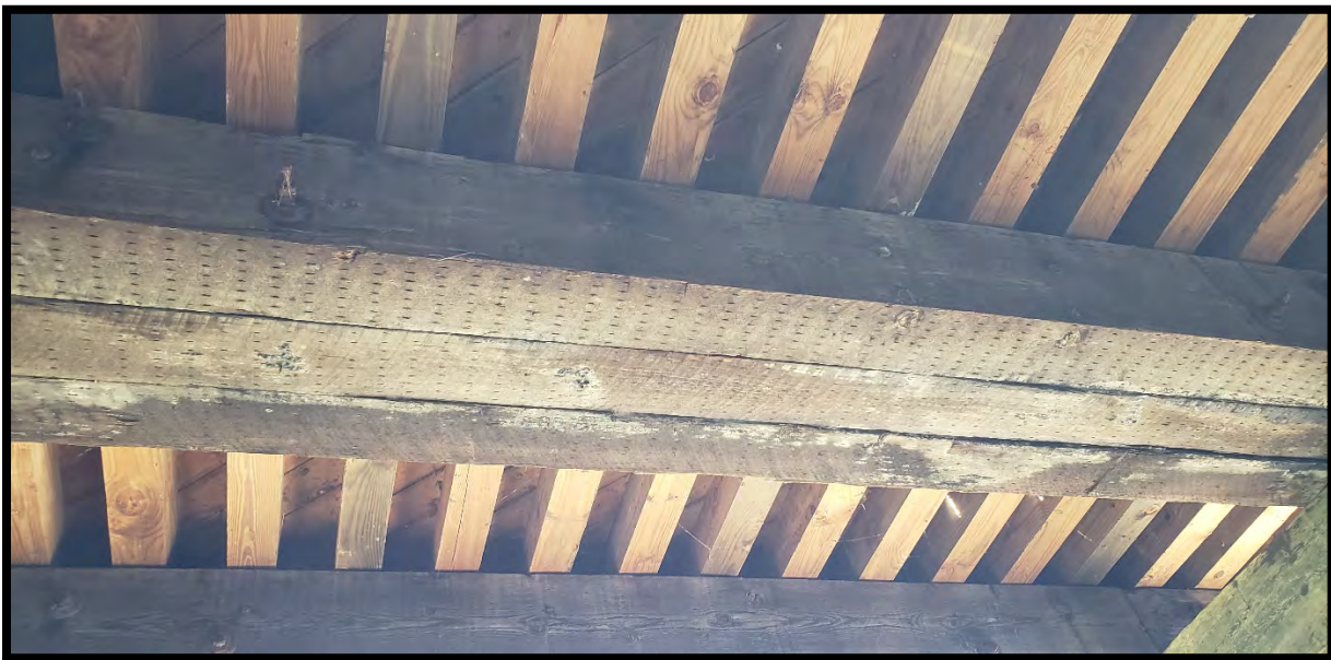
Superstructure-Timber Stringers and Floor Beams
