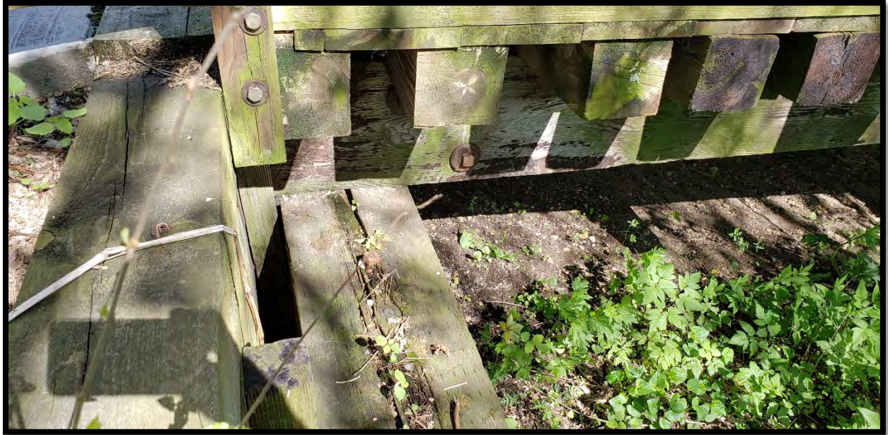
South Abutment-Pile Cap Deterioration
