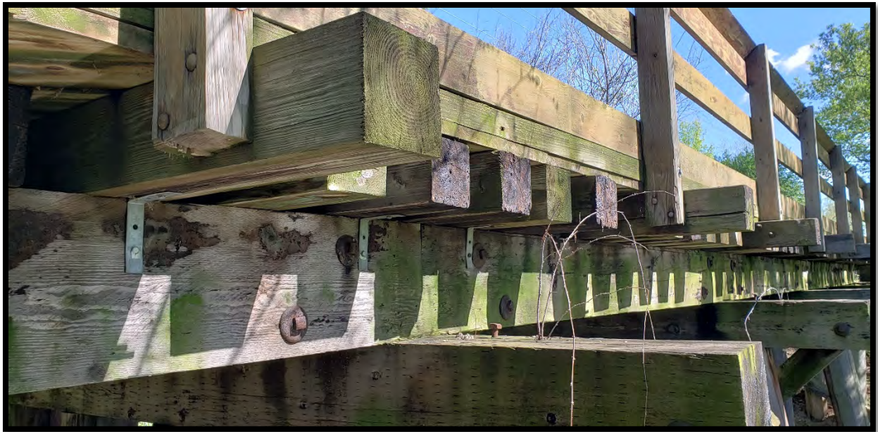
Timber Railing fastened to cantilevered Floor Beams
