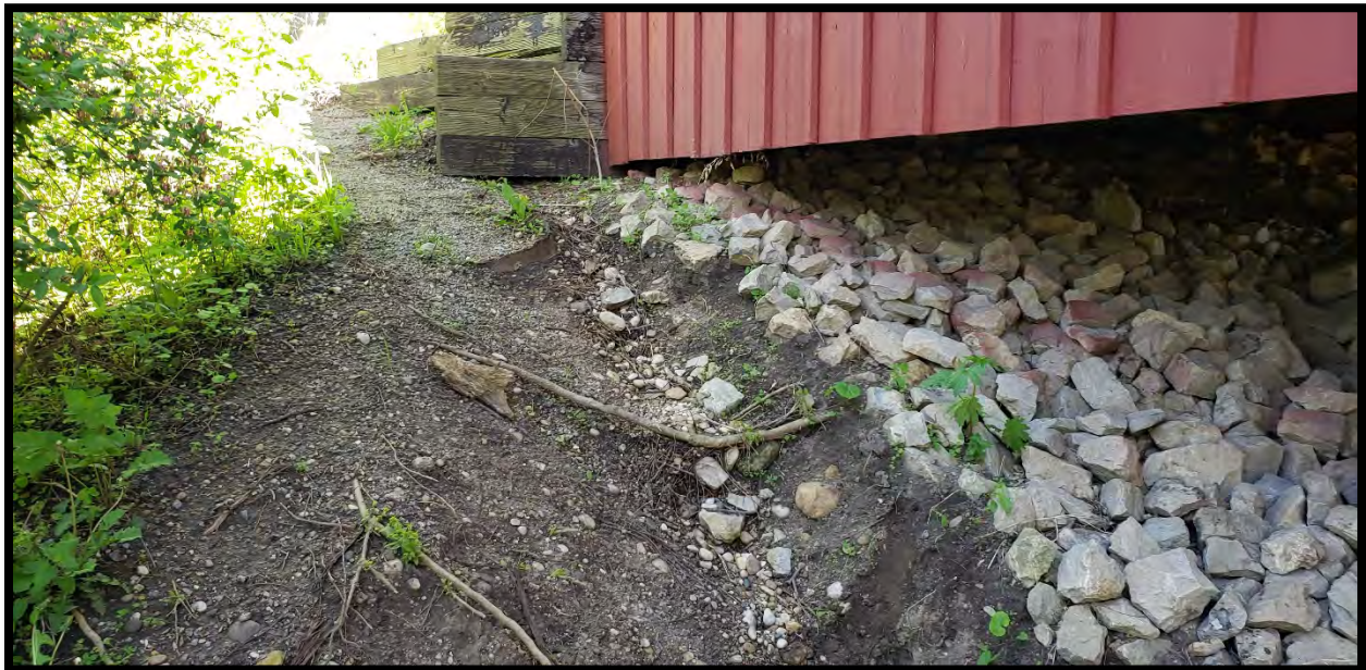
Slope Erosion-NW slope
